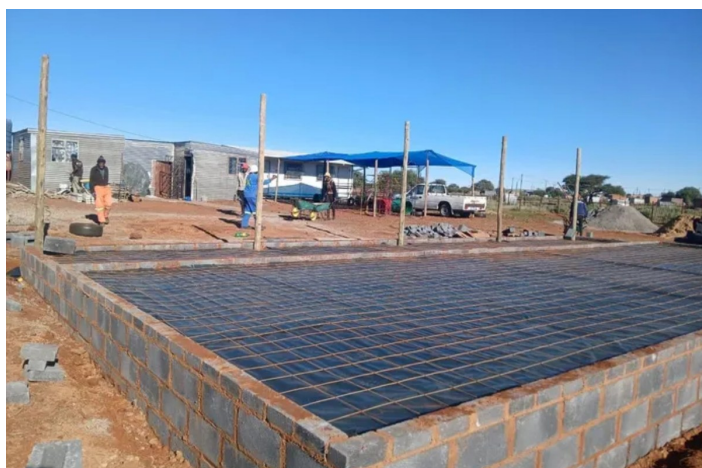
Ground was broken on May 4 for the new Reaiteka Early Childhood Development centre in Maruping Village near Kuruman. The project is expected to be completed in July and will provide safer, improved learning spaces for young children in the rural community.
