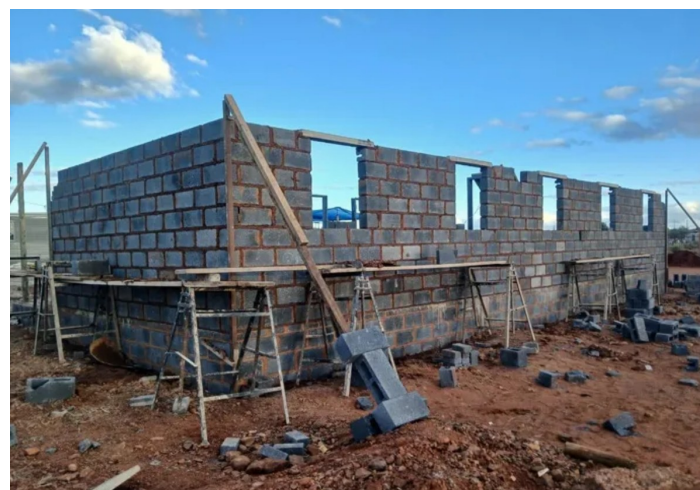
Maruping Village, about 15km from Kuruman, is set to receive a brand-new brick-and-mortar building at the Reaiteka Early Childhood Development centre through a partnership between the Santa Shoebox Project, the Centre for Early Childhood Development, Breadline Africa and Kathu Solar Park.
